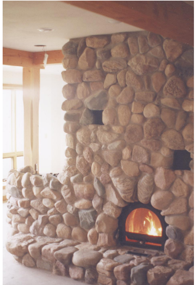
Above: Envirotech masonry heater module. Stone for the facing was gathered onsite.
